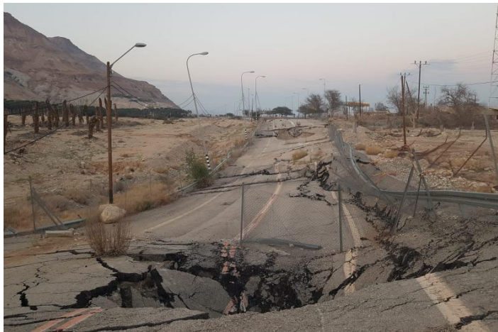
Fig. 5 – A section of the Jerusalem-Eilat road near Ein-Gedi (Dead Sea shoreline), that was recently abandoned due to opening of sinkholes.
